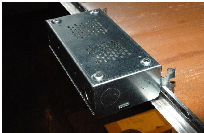
Mounted to T-Bar using the integral T-Wings
